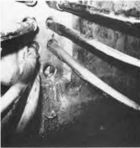
Figure 26.27 MV underground feeders in concrete duct.
