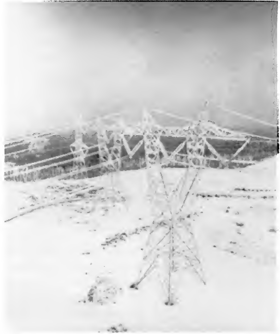
Figure 25.6 During winter, steel towers must carry the combined weight of conductors and accumulated ice. (Courtesy of Hydro-Québec)
