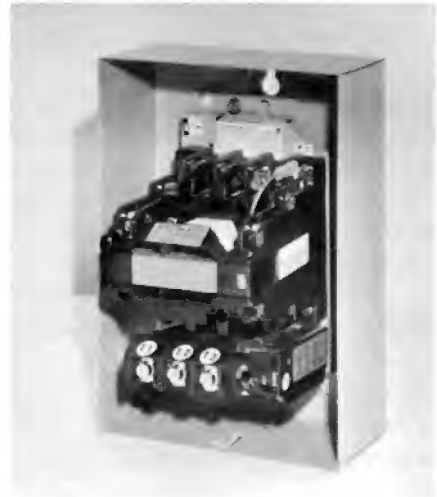
Figure 20.16a Three-phase across-the-line magnetic starter, 30 hp, 600 V, 60 Hz. (Courtesy of Klockner-Moeller)
