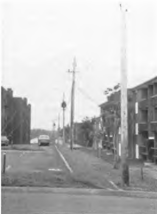
Figure 26.28 MV aerial feeder serving a residential district.
