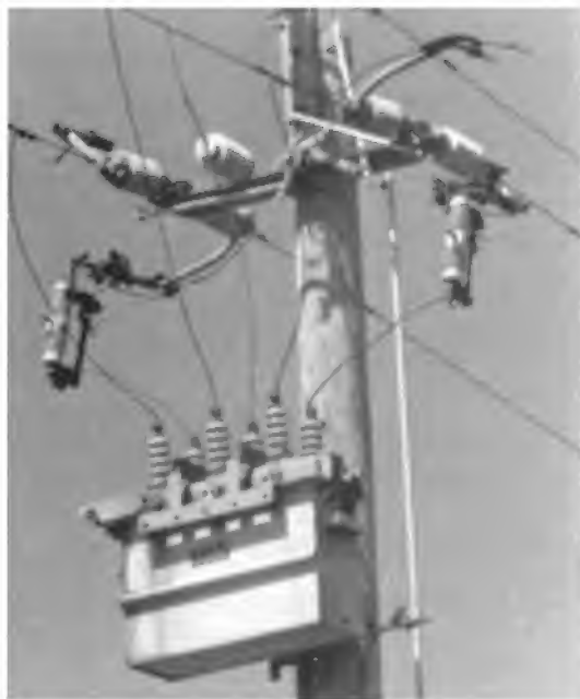
Figure 26.33 Automatic recloser protecting a 3-phase feeder.
