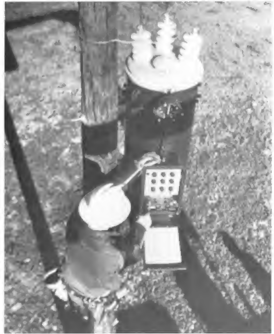
Figure 26.29 Automatic tap-changing autotransformer maintains steady voltages on long rural lines. (Courtesy of General Electric)
