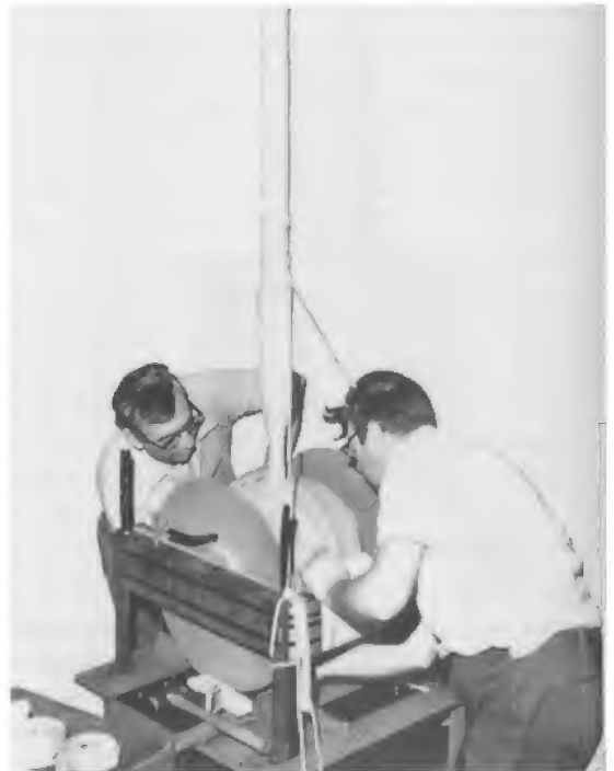
Figure 11.15 Current transformer in the final process of construction. (Courtesy of Ferranti-Packard)
